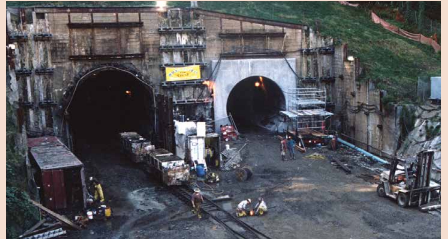
Westside MAX tunnel east portals, 1995
