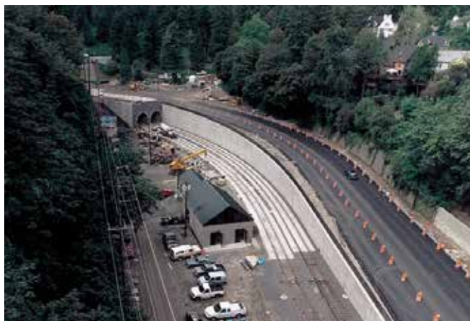
Westside MAX tunnel east portals, 1997
