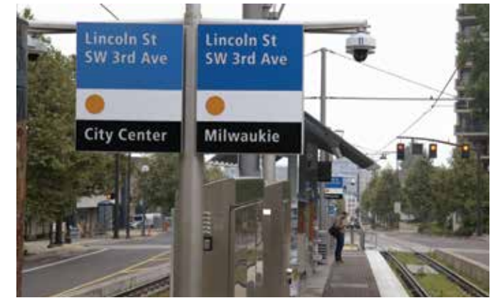
Orange Line MAX platform cameras, 2015
