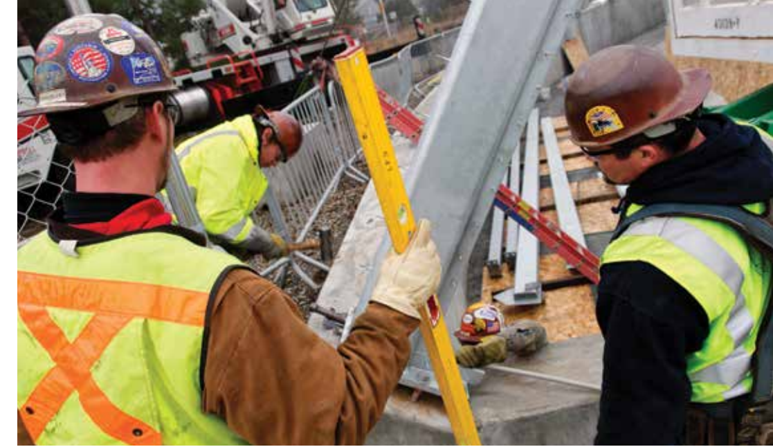
Construction workers on MAX Green Line, 2009
